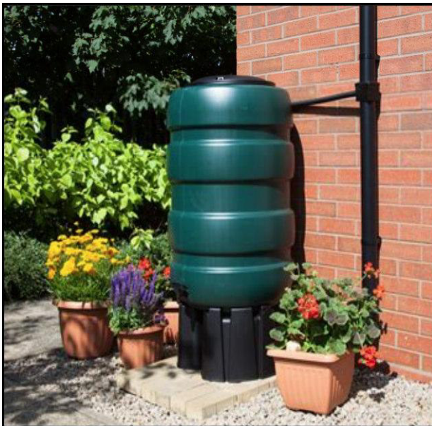
Figure 6: Rainwater Butts (Ciria 753, Figure 18.5)
